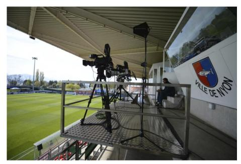
Positioned in the main stand and situated exactly on the halfway line, these cameras must be covered and must face away from the sun. Space should be provided for at least two cameras on a platform at least 4m long and 2m wide. The cameras must have a full and clear view of the whole pitch, and it must be possible to use them unaltered, i.e. without applying side viewfinders.
